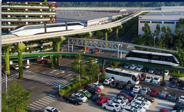
SkyRail (left) and SkyShuttle (right) servicing Shenzhen, China
